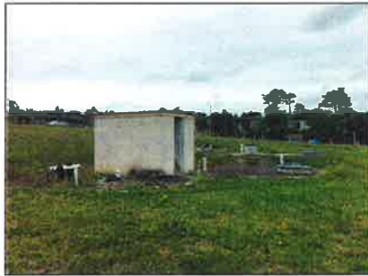
Photo 2: Former wastewater treatment plant
